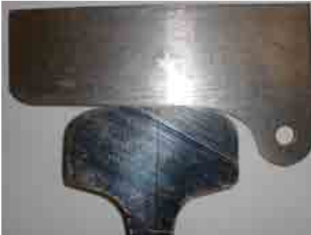
Correct head shape and proper wheel to rail contact after grinding
